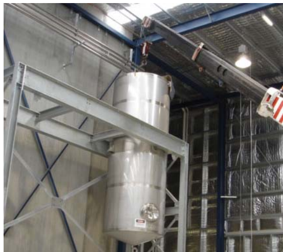
Site upgrades increase existing production
