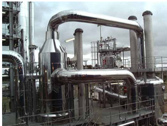
Site upgrades increase existing production
