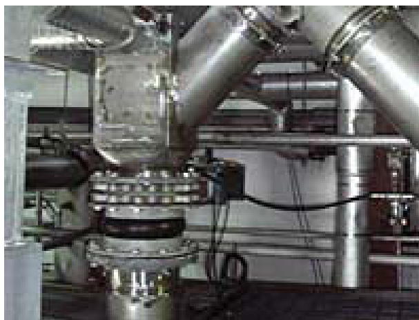
Site upgrades increase existing production
